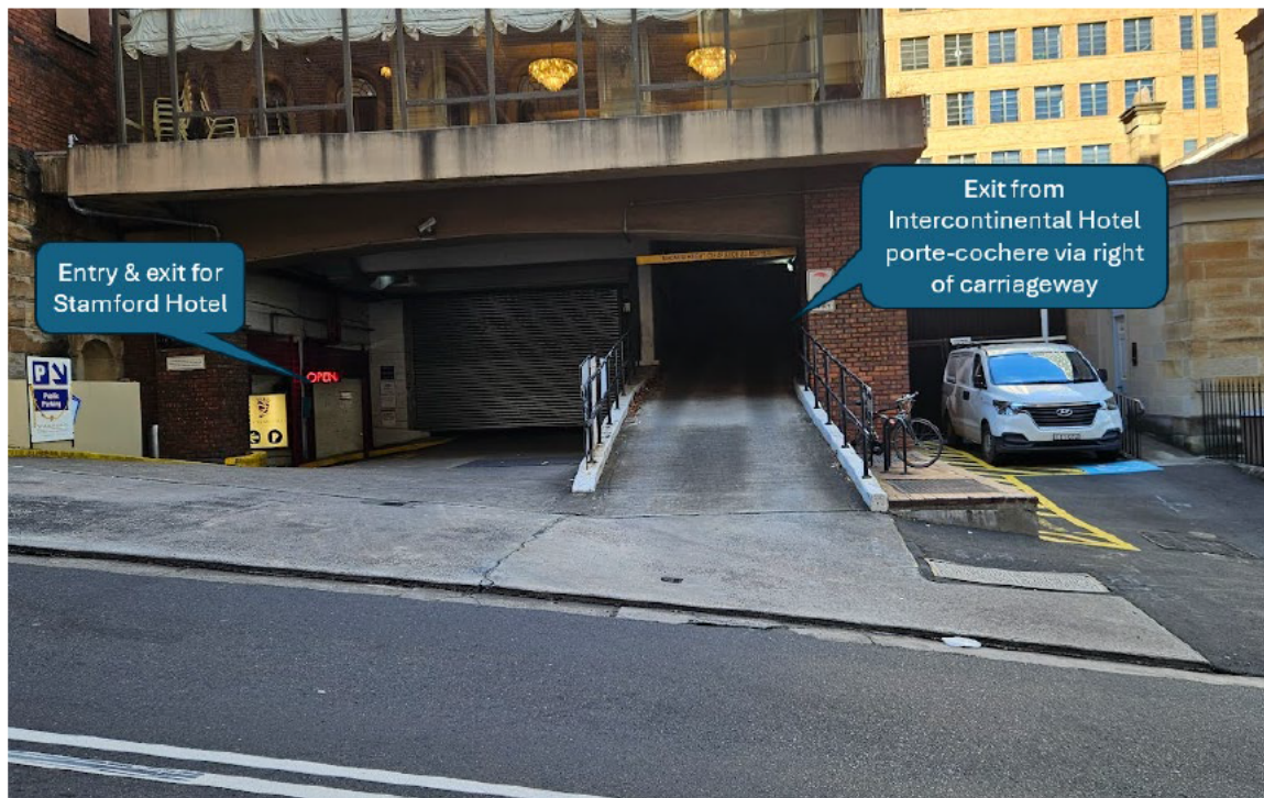
Figure 3 Existing vehicle egress from right of carriageway
